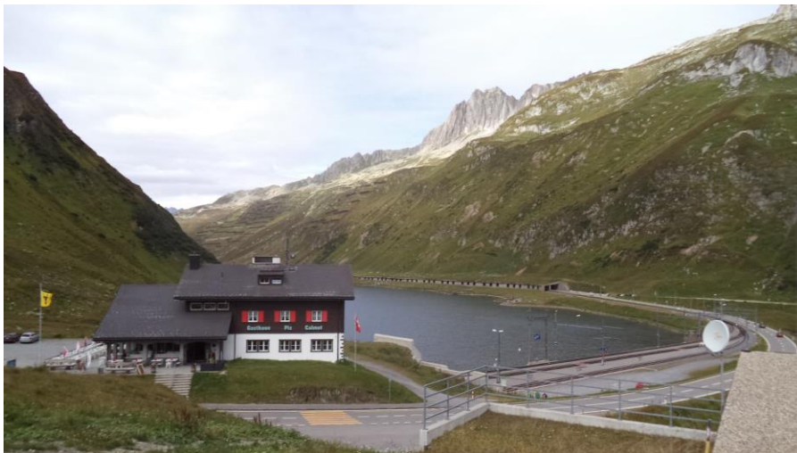
Oberalppass train station.
