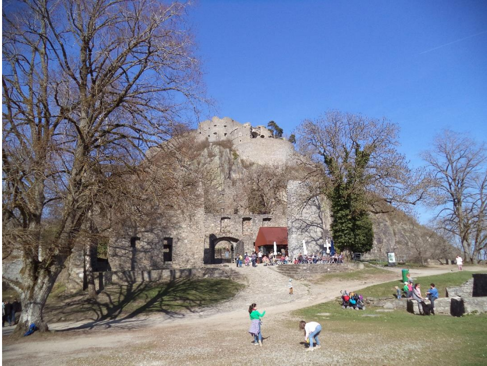
The park at the entrance gate to the fortress; the fortress is visible in the background at the top.
