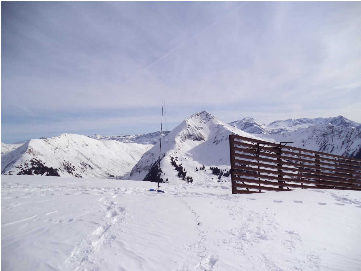
This metal snow fence is the only support in the activation zone.
